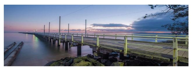
The iconic Urangan pier was built between 1913 and 1917 as a cargo-handling facility originally to facilitate the export of sugar, timber and coal. The original length of the pier was a total of 1107 meters, however it was closed in 1985 and 239 meters of it was demolished. Due to public outcry 868 meters of the pier was left and has since been fully restored.
